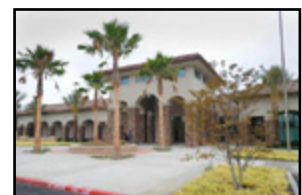
03 South Los Angeles Sheriff's Station
