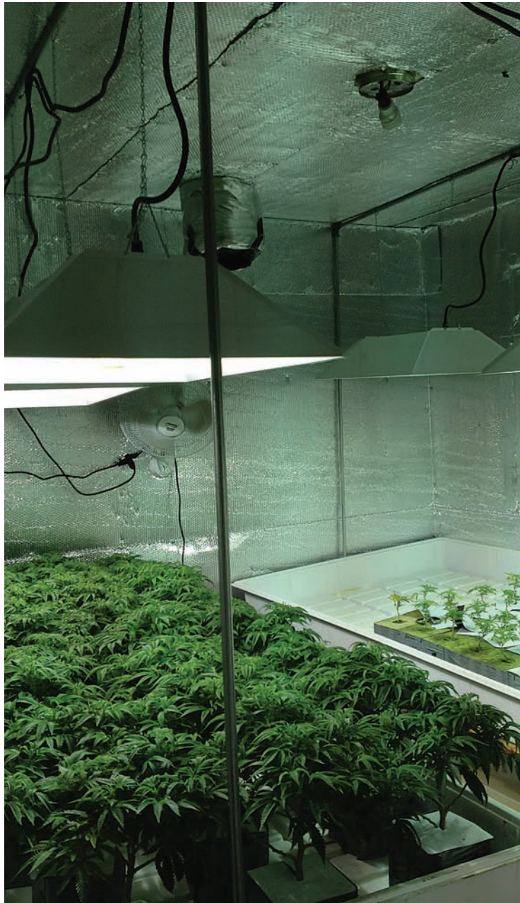
One of 4 rooms converted into grow rooms. Notice the sophisticated and elaborate lighting and HVAC systems hanging from the ceilings.
