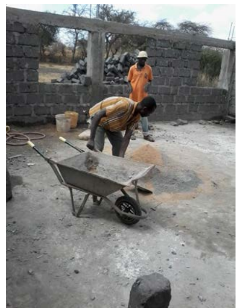
Workers building the future.
